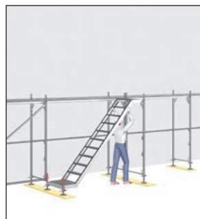
Fig. 64: Insertion of platform stairway
